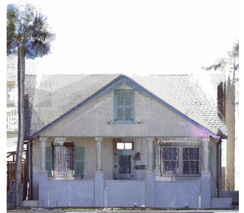
Coquina/Slab on Grade Foundations
